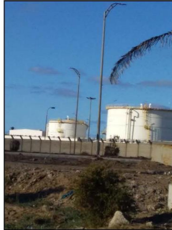
photo.2. gas tanks in methanex plant Damietta port Source: field study, 17 oct.2020
